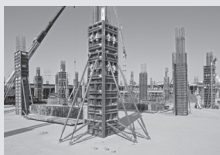
Column formwork
