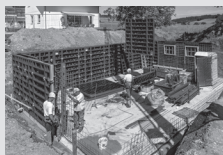
Wall formwork
