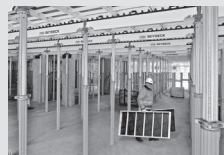
Slab formwork
