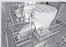
Working scaffolds industry
