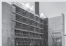
Working scaffolds construction
