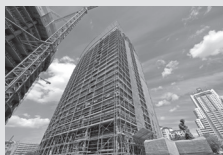
Facade working scaffolds
