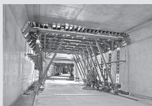
Tunnel formwork
