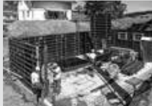
Wall Formwork
