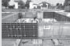
Wall Formwork
