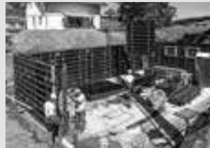
Wall Formwork
