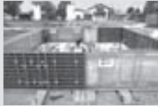
Wall Formwork
