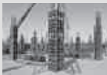
Column Formwork
