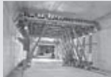
Tunnel Formwork
