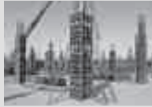
Column Formwork
